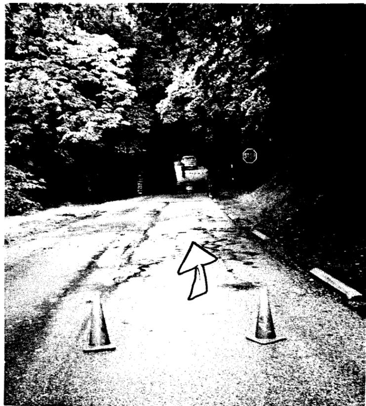
The heavy rains of June 18 rose to the level indicated by the arrow, carrying mud, silt and a huge tree trunk two feet in diameter, through the tunnel. Maintenance workers had to remove the mud before the tunnel could be reopened to traffic.
