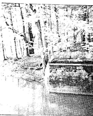
4. The village recently cleared this 24 inch culvert under Indian Hill Rd. at a cost of \$972. Silt filled channel on private property south of Indian Hill Rd. was not cleaned and water flow remains impeded.
