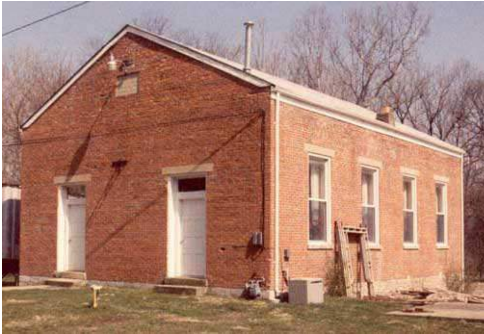
The brick Miami Baptist Church in Montauk was built in 1847.
