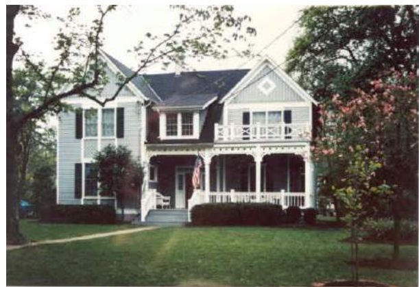
313 Oxford Avenue was moved from Rugby Avenue in the 1920s. 1998 photo
