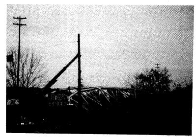
Workers next removed all braces except for the two end pieces. To make the structure fall, notches were cut in the two end pieces.
