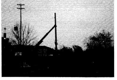
Finally, a cable was attached to the center of the steel arch span: and, when two giant buildozers pulled, the structure neatly folded upon itself and fell down into the river.
