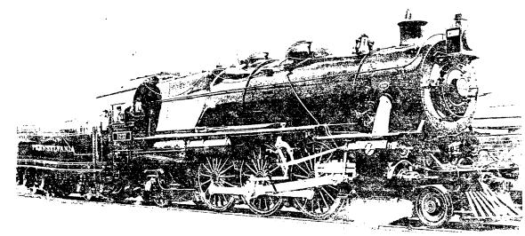
This locomotive is typical of the engines that passed through Terrace Park in the neggay of the Pennsylvania Railroad. It was known to railroad buffs as a 4-6-2, having four small guiding wheels at the front, six main driving wheels, and two small trailers under the cab.
