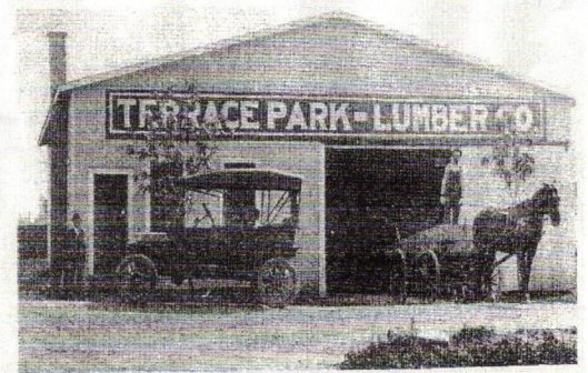
The lumber company in early days, with the founder at far left.
